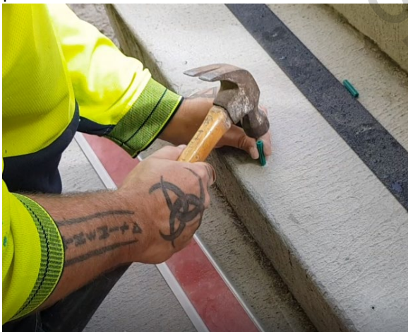
Insert green plug and hammer in
