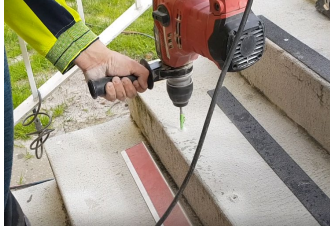
Using the countersunk holes as a guide, drill a much larger hole to accommodate a plug.
