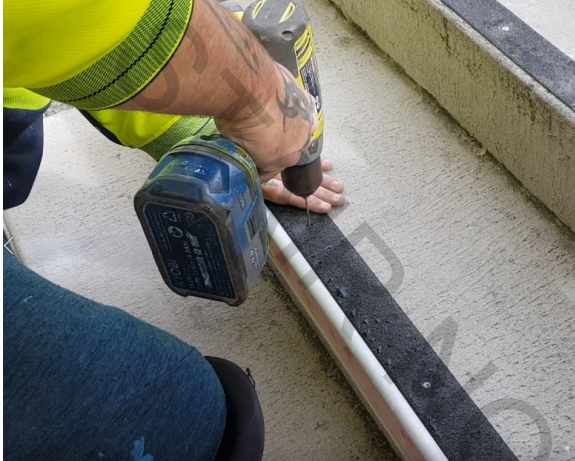
Using pre-drilled holes in the FRP strip, drill a pilot holes
