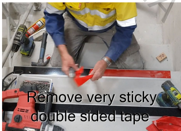
Gently position nosing on step edge if the adhesive bleeds wait for it to dry and then scrape off
