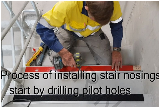
Drilling a larger hole to countersink the screws so they don't sit proud
