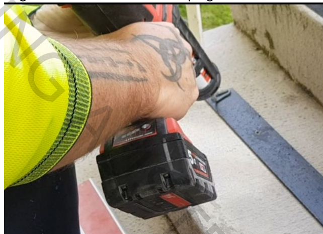
Using the countersunk holes as a guide, drill a much larger hole to accommodate a plug.
