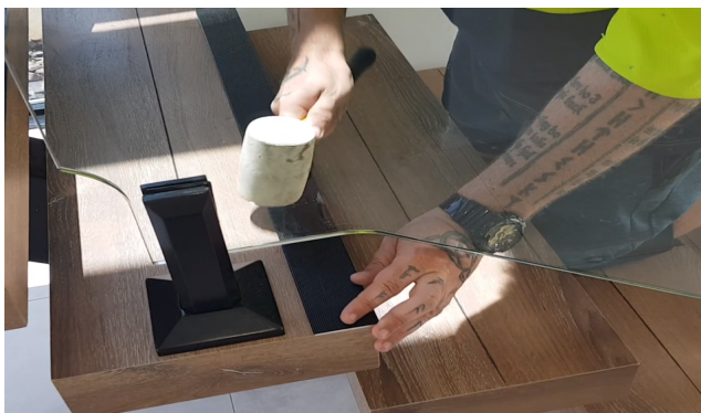
Using a rubber mallet tap nosing on step edge
