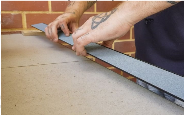
Gently turn stair nosing over, and position on edge of step.
