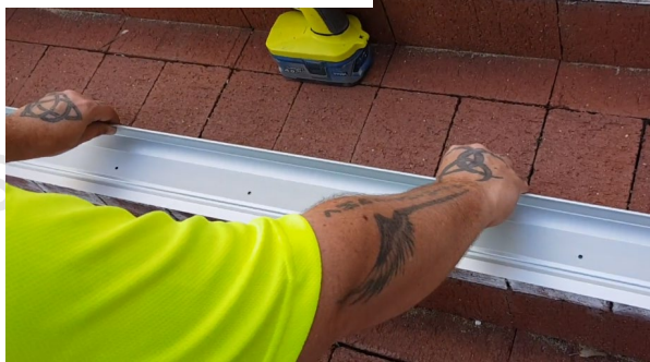
Place stair nosing on step edge upside down.
